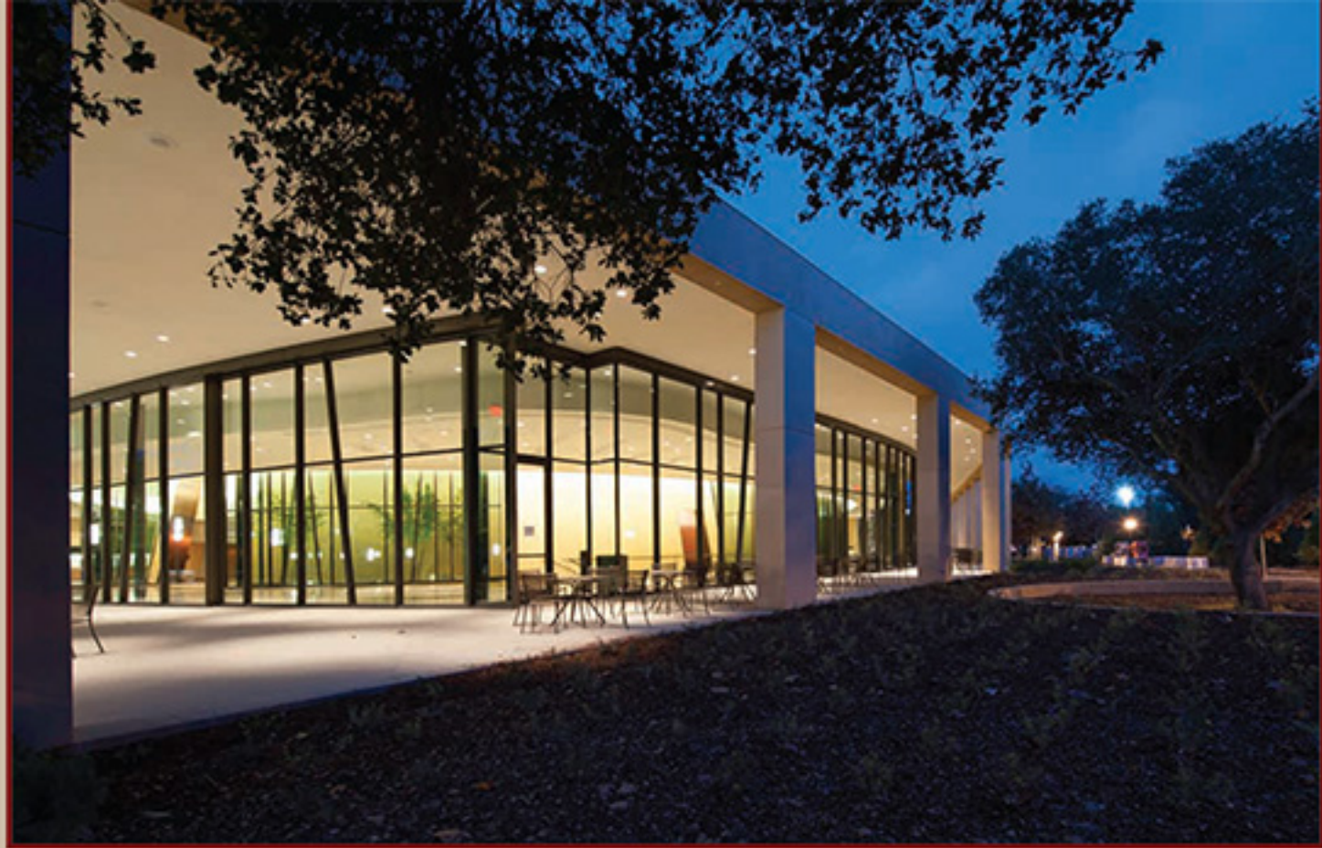
An exterior view of the lobby at dusk.
